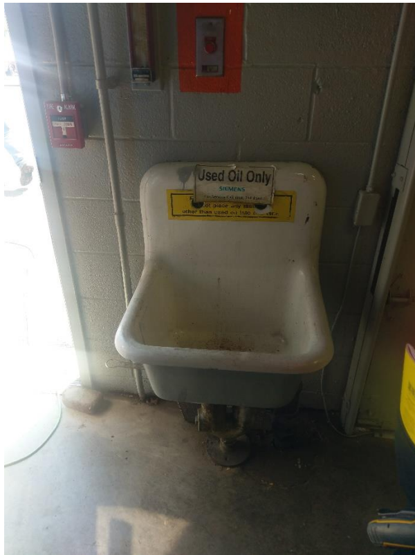
Used Oil Sink to Exterior UST (Auto Mechanic Shop)
